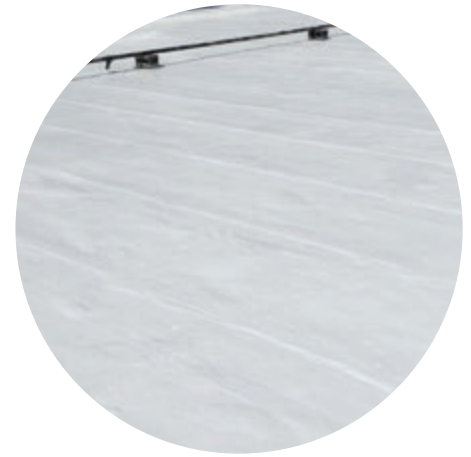
*MonoTop finished product on roof
