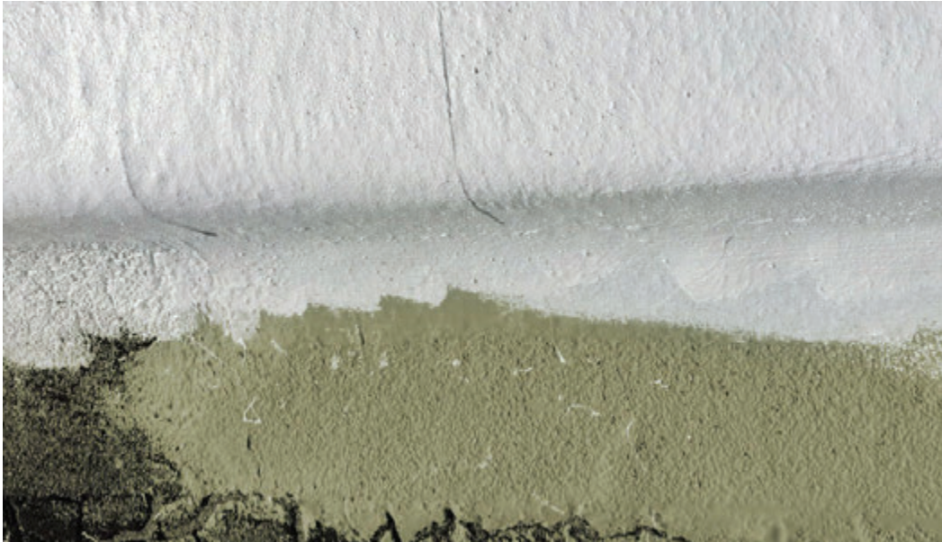
*MonoBase (tan) with MonoTop being applied.
