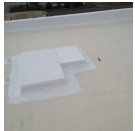
AguaBase with MonoTop flashing detail
