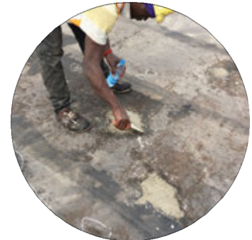
AguaPlus for repair and leveling
