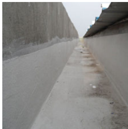
AguaBase: providing watertight integrity to gutters between roof panels
